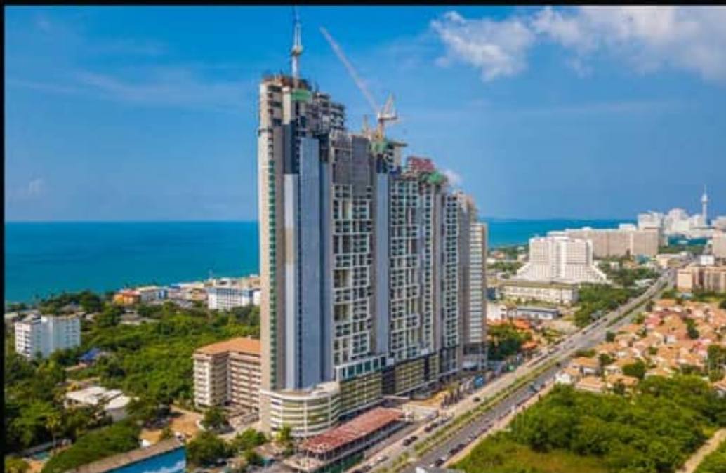
Construction as of November 2018
